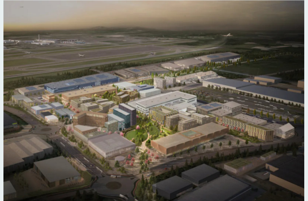
Gardermoen, Oslo Airport in Norway
