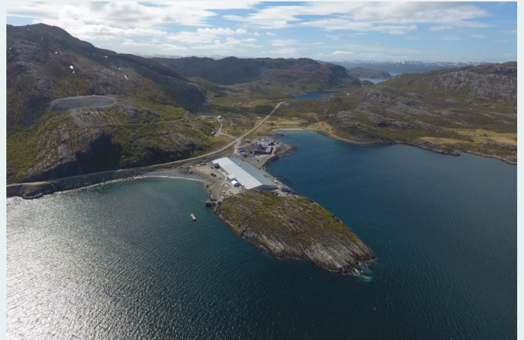
Adamselv smolt facility in Finnmark
