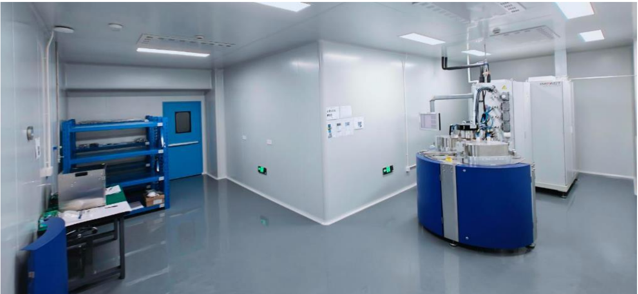
The coating system transferred from Sweden installed at the Coating Service Center China, for coating of waveguide antennas for Waveland Technology.
