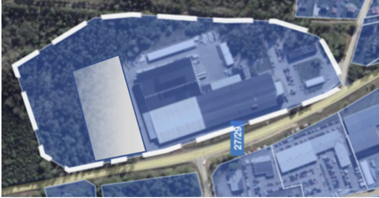
Scratched surface shows possible area for expansion
