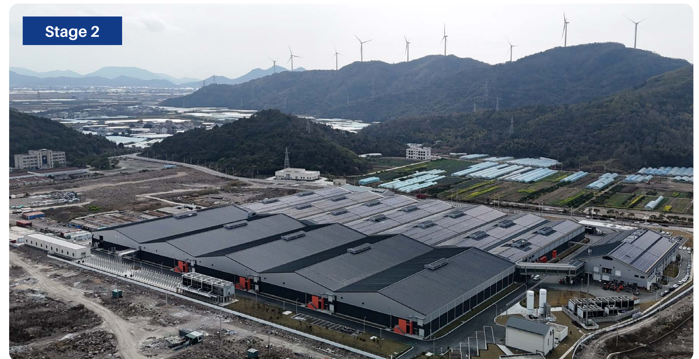
Gaotang production facilities March 2026
