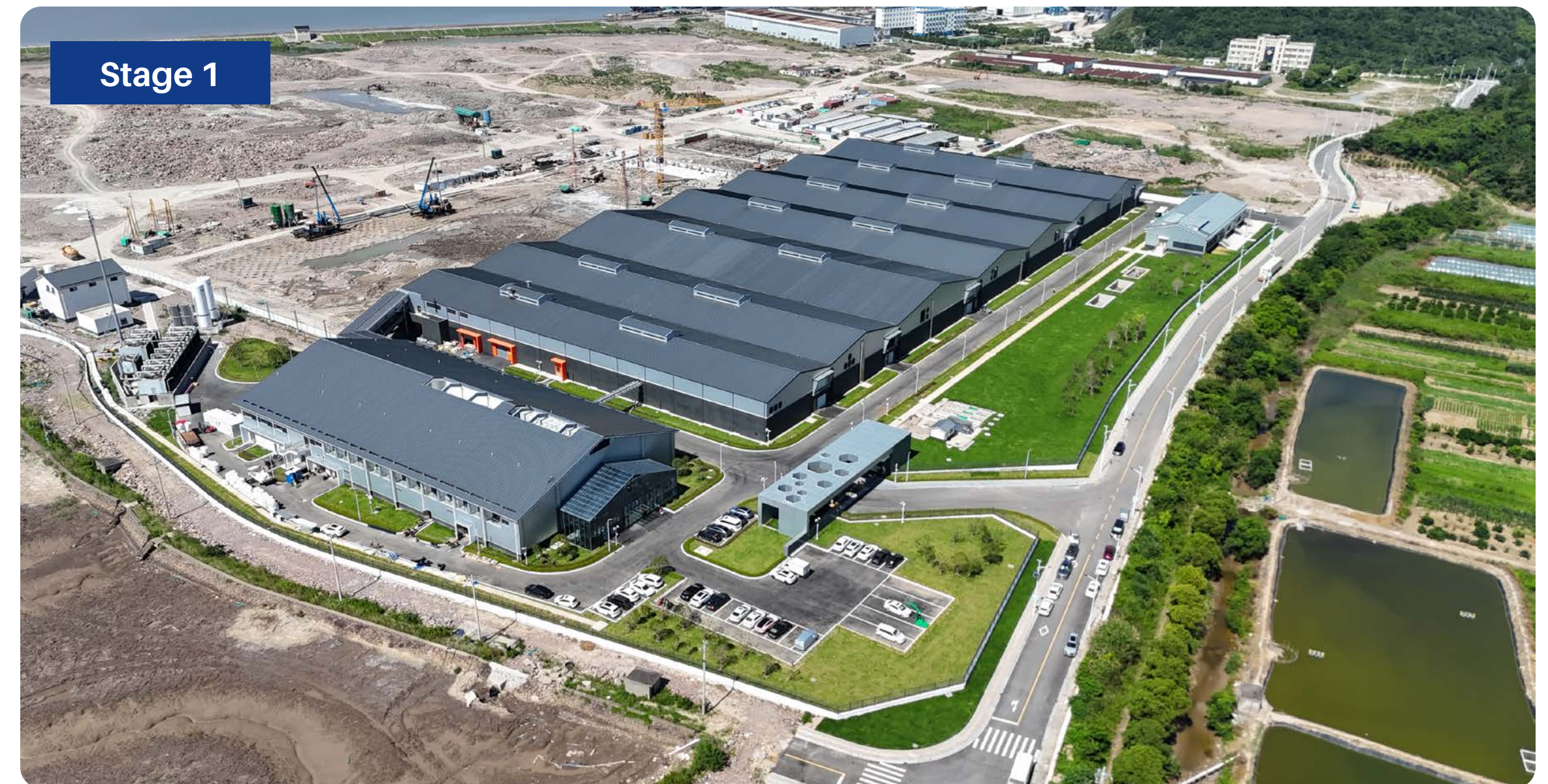
Gaotang production facilities July 2024
