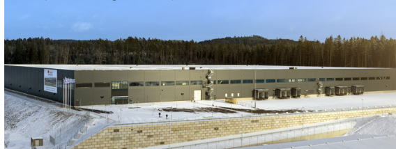
Nelly's warehouse in Borås, completed during the first quarter.
