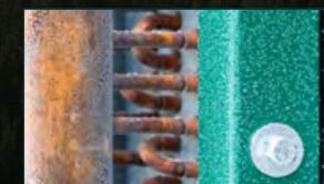
Cover: Detailed image from our Bredhälla BESS (Battery Energy Storage System) energy storage project in Sweden.
