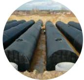
increasingly common problems such as floodings caused by increased rainfalls due to climate change. Such tanks are mainly used in commercial areas with large, paved surfaces where water drainage, storage and cleaning solutions are required.
