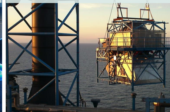
Statfjord C – Installation of waste heat recovery unit
