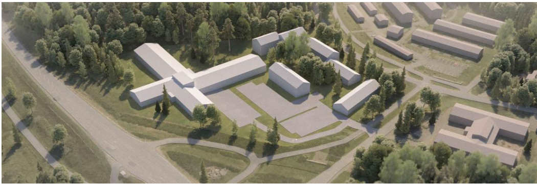
Care property portfolio in Finland – New build project (Q4 transaction)
