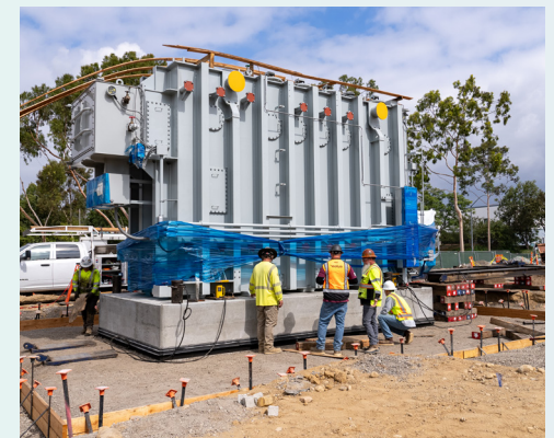
Delivery of a transformer to the project site.
