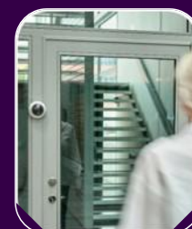
Physical access and visitor management
