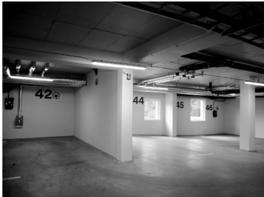
Parking structure with EV charging capabilities, Vårbergstoppen, Vårberg
