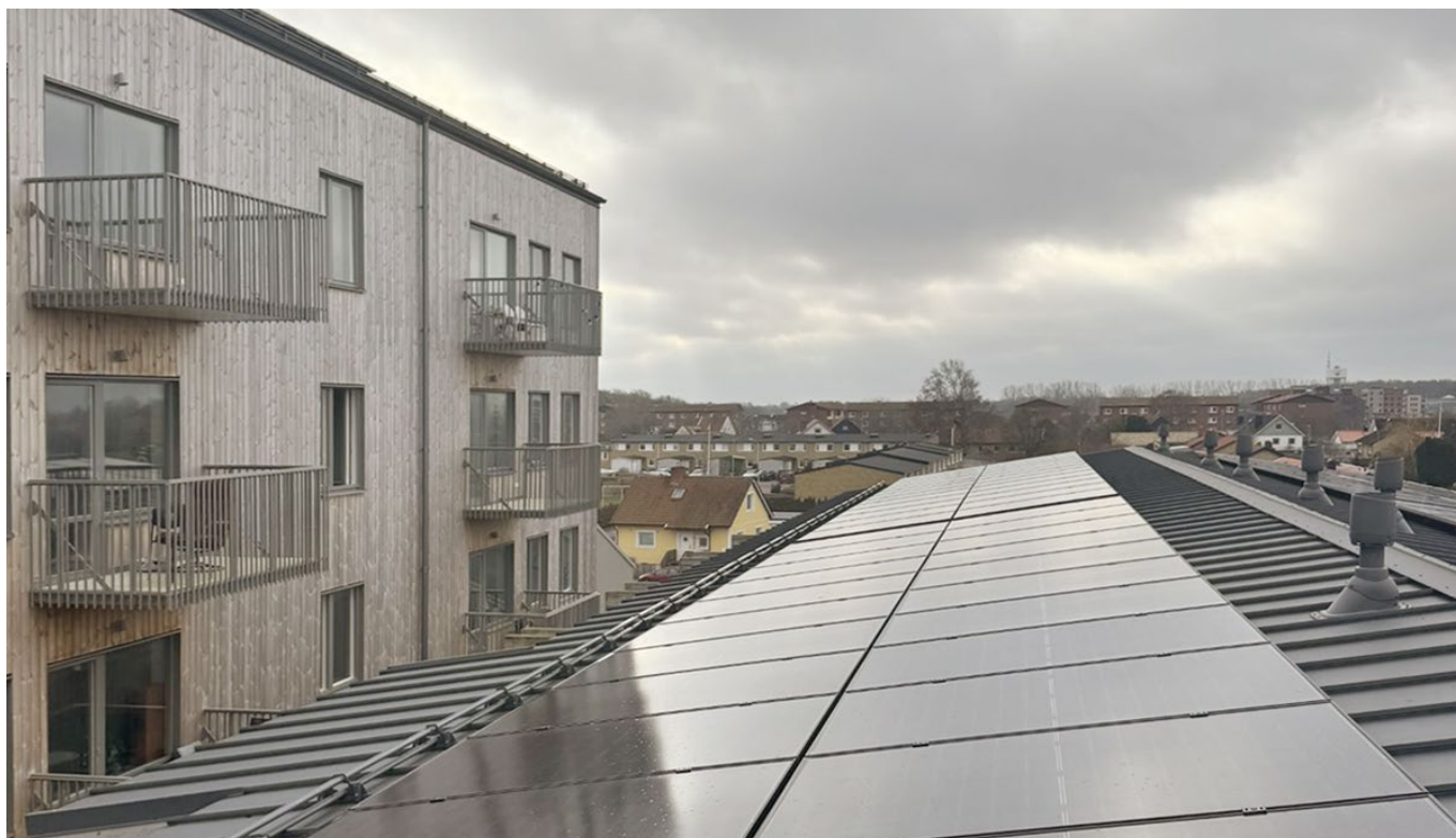
Solar panels were installed at KlaraBo properties in Svalöv.
