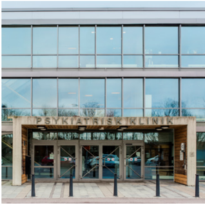
Skåne (Malmö, Lund and Helsingborg) Health care/Higher education/Justice Number of property units: 4 Lettable area: 86,300 sqm Number of employees: 1 (Establishment of the organisation in progress)
