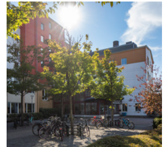
Vänersborg, Lasarettet 2 Office
