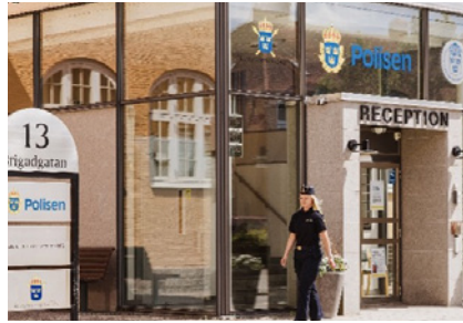
Linköping, Smedstad 1:21 (Garnisonen), National Forensic Centre, Swedish Police. Completed Q4 2020.
