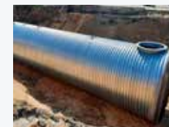
Fire water tank
