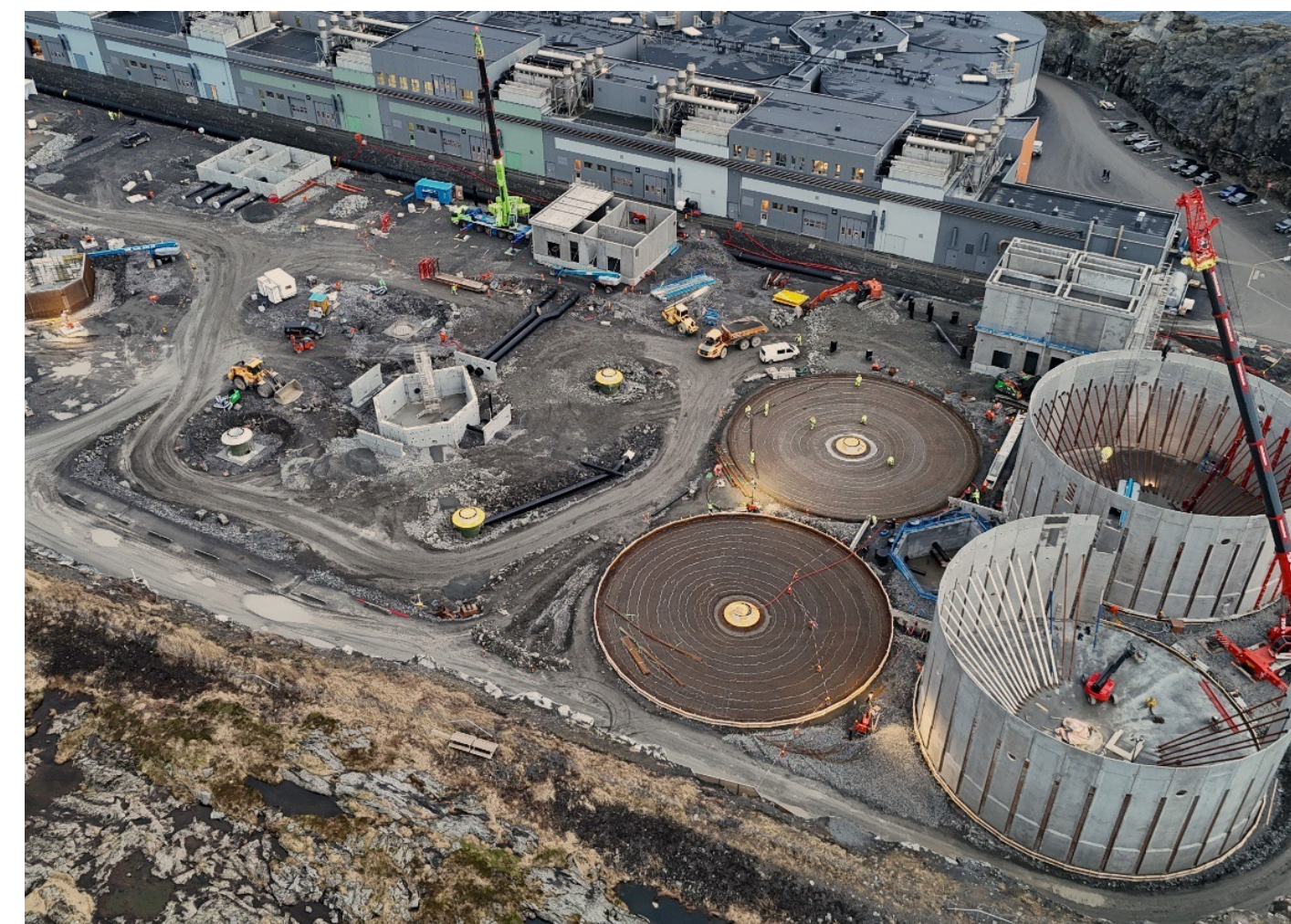
Tank installations well underway (February 2025)
