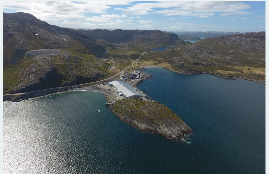
Adamselv smolt facility in Finnmark
