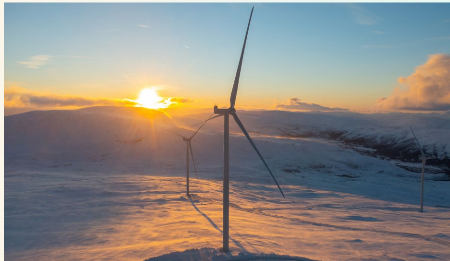
The Øyfjellet Project was completed and handed over to its owner, Øyfjellet Wind AS, in March 2023. The facility comprises 72 wind turbines with annual electricity generation of about 1.3 TWh. The electricity provides Alcoa's production facility in nearby Mosjøen with renewable electricity, enabling Alcoa to make extensive investments in the facility.
