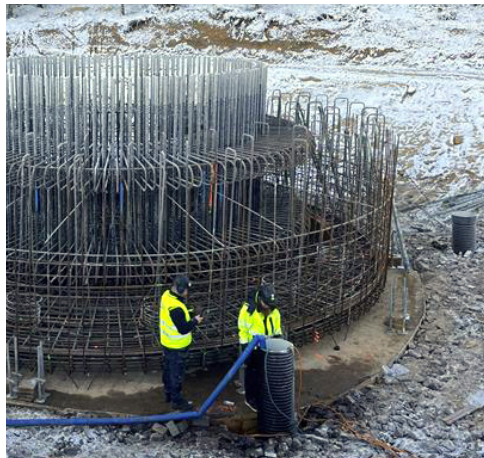
Casting a foundation for a wind turbine.
