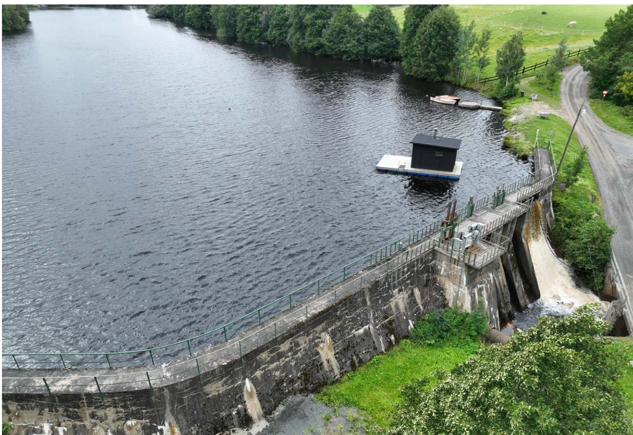
Klerebo dam, Klerebo power plant in Bankeryd.
