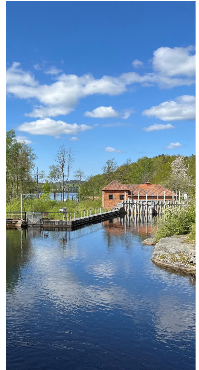
Ålgårda power station in Kungsbacka
