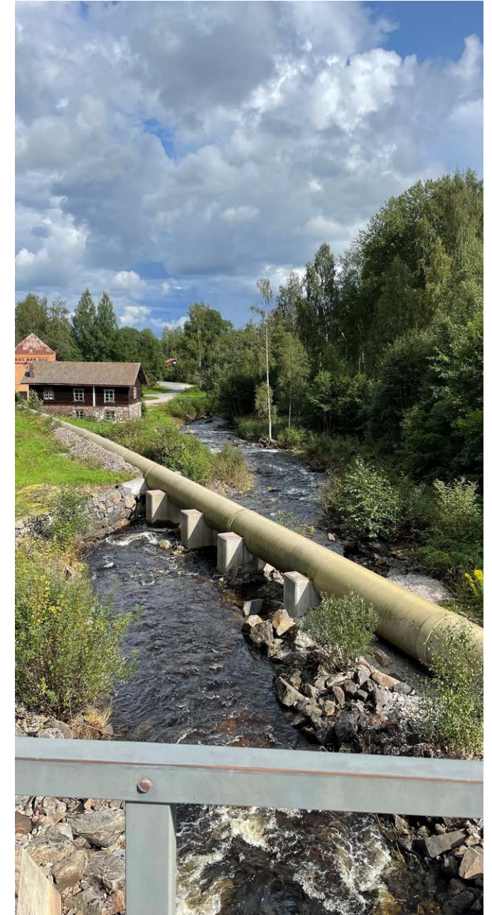
Gopa power plant in Sägmyra, Falun
