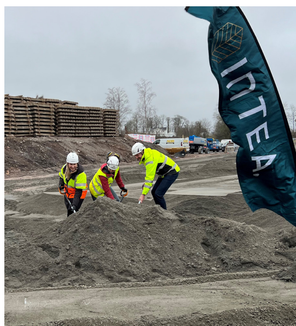
Breaking ground for a new train depot in Falköping.
