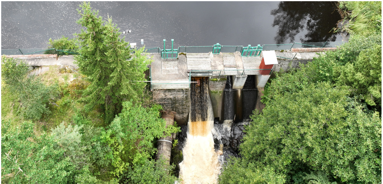
Hulebodammen, Hulebo power plant in Bankeryd.
