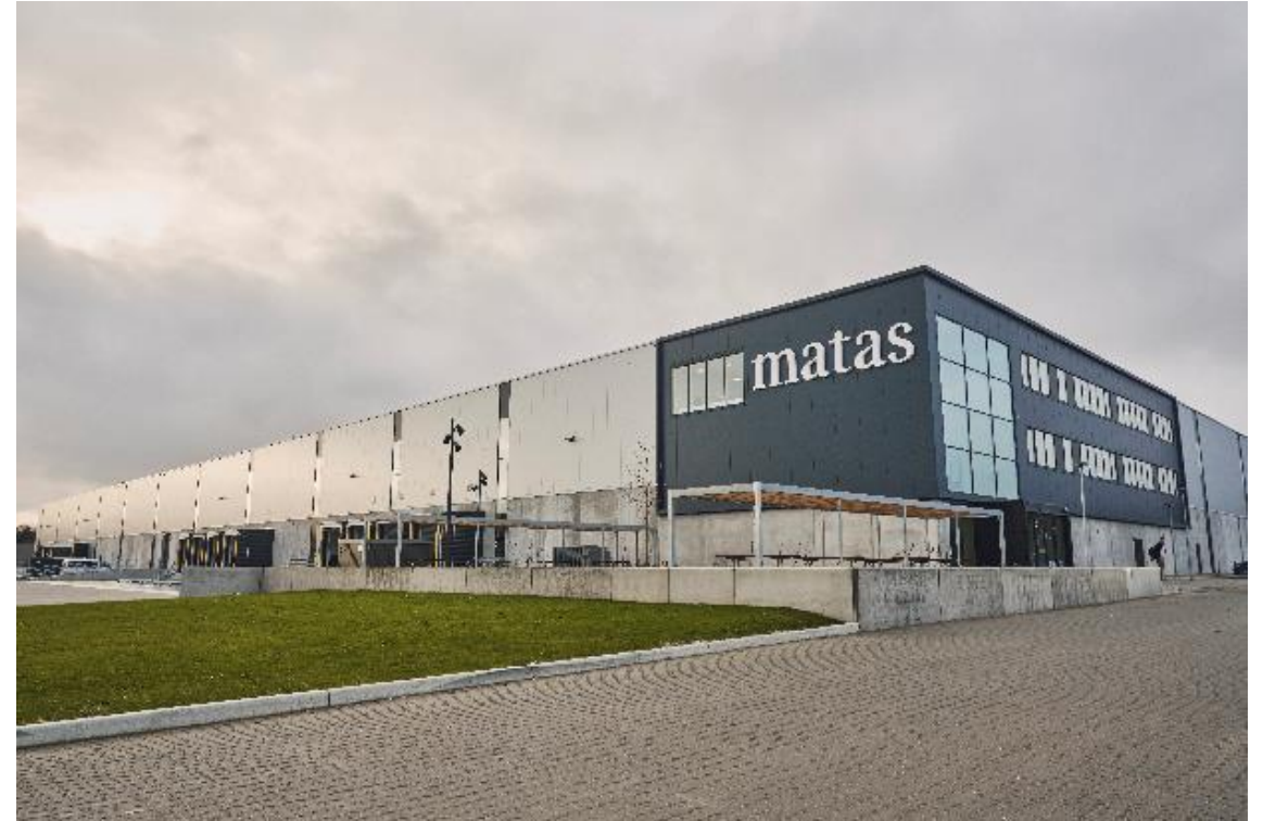
Matas automated logistics center (MLC) in Lyngø, outside Copenhagen
