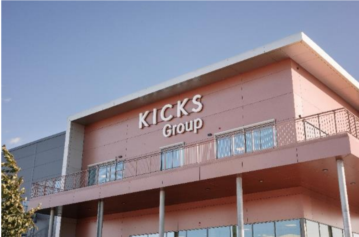
KICKS automated logistics center (KLC) in Rosersberg, outside Stockholm
