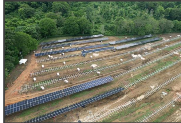
Planeta Rica Colombia Overall progress: 65% Module Installation
