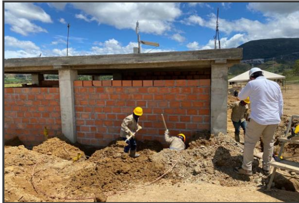
Los Girasoles Colombia Overall progress: 72% Module Installation
