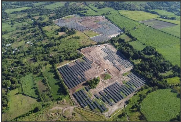
Santa Rosa & Villa Sol El Salvador Overall progress: 88% Module Installation
