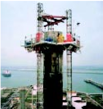
A work platform from Alimak Hek is used to dismantle a chimney in Rotterdam harbour.
