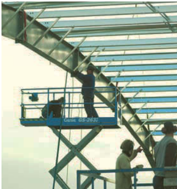
Acquisition of Astron has made Lindab the market leader in prefabricated steel buildings in Europe.
