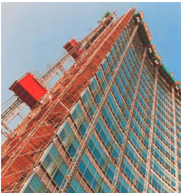
Equipment from Alimak Hek is used in the construction of the Zuidtoren office building in Hoofddorp, the Netherlands.
