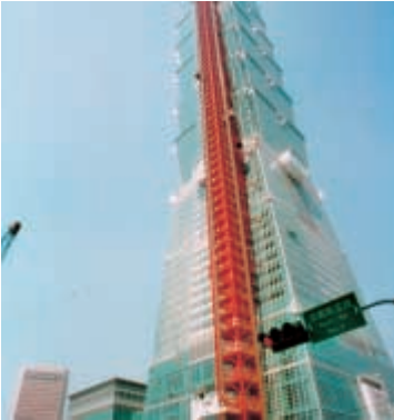
Equipment from Alimak was used in the construction of the world's tallest building, the Taipei Financial Centre in Taiwan.
