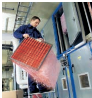
Changing a Hi Flo air filter, Camfil's largest product.
