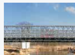
Temporary and permanent bridges
