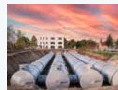
Oil and sand separator
