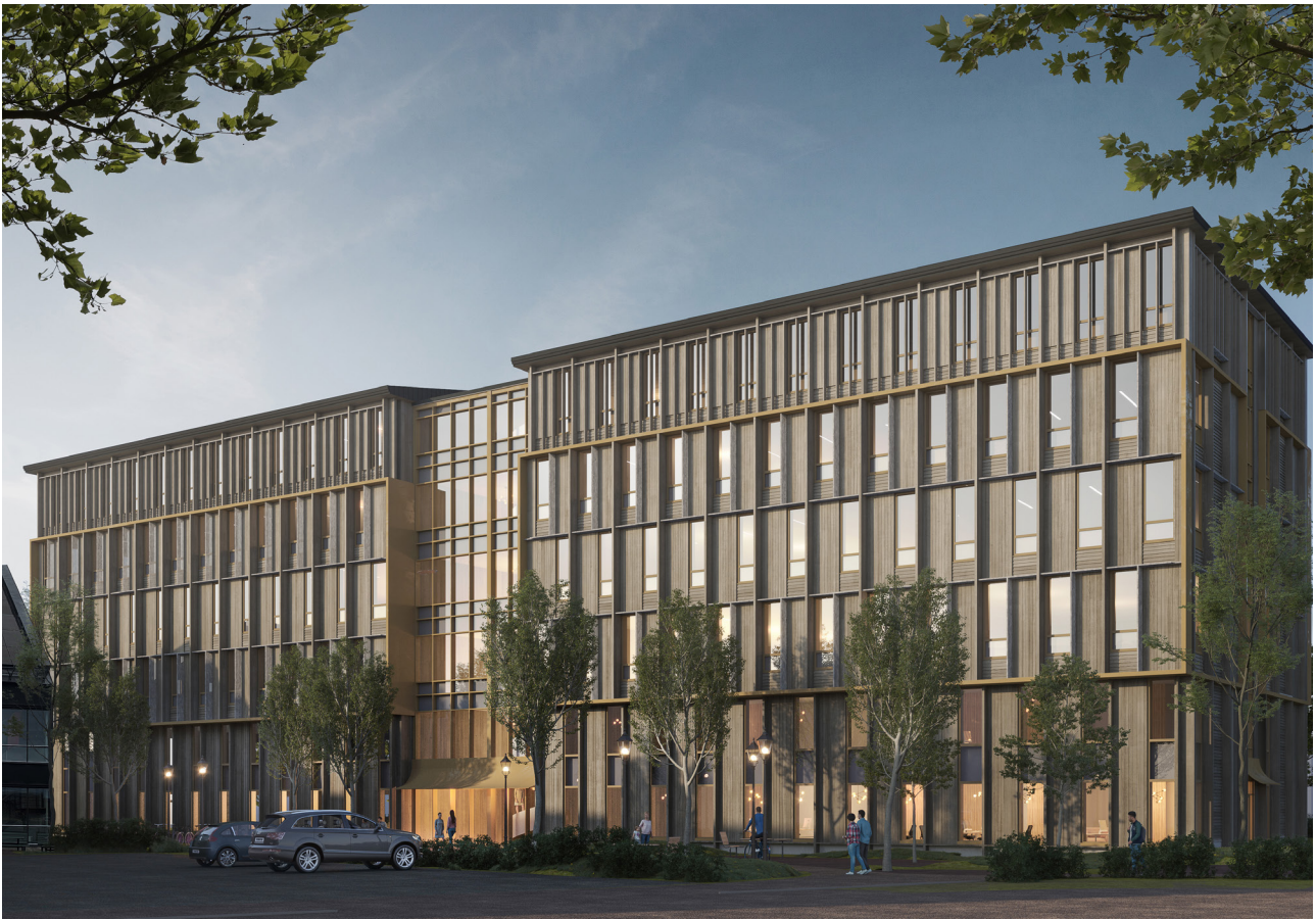
Intea's new wooden building is under construction on the in Östersund campus
