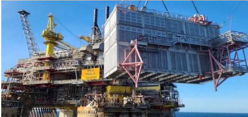
Troll West Electrification
