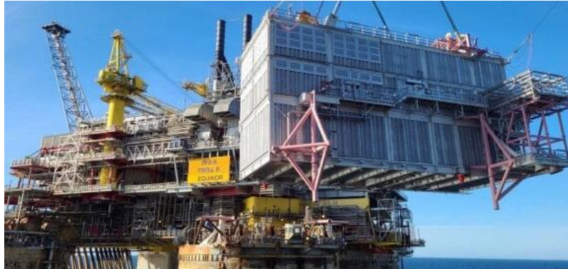
Troll West Electrification
