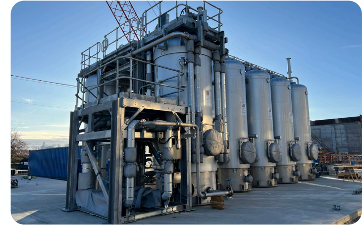
THP installed at Blue River wastewater treatment plant in Kansas City, Missouri, USA
