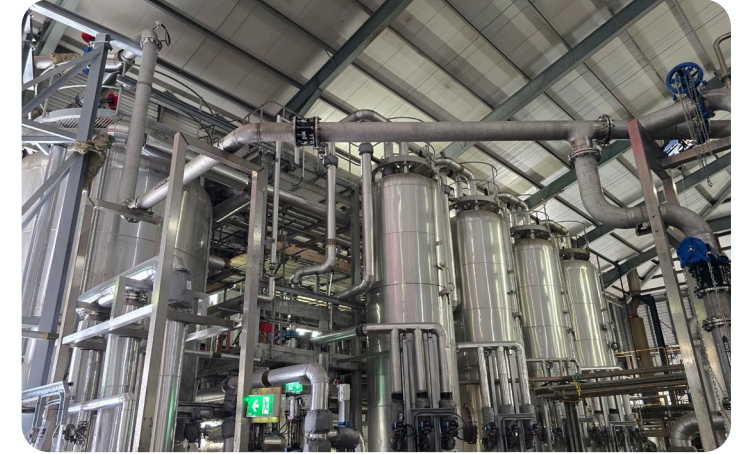
Upgraded THP stream at Ringsend in Dublin, Ireland
