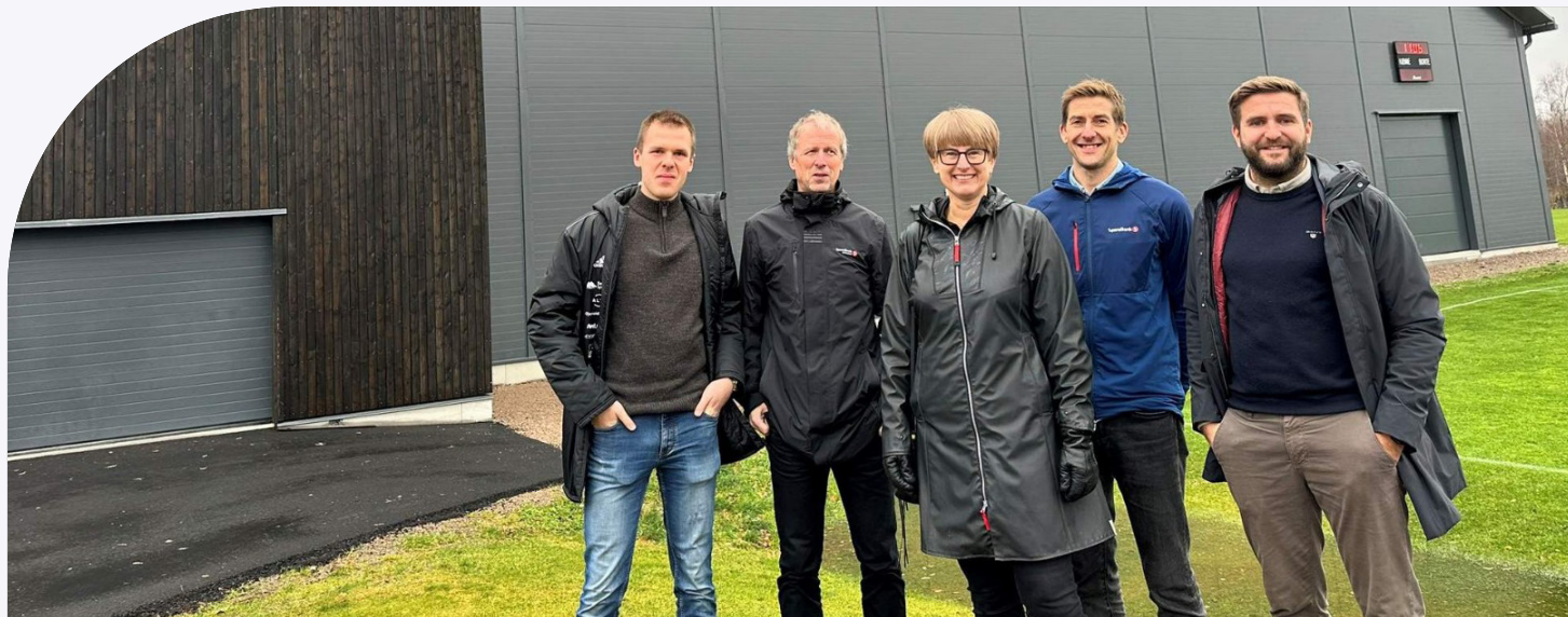
Bankhallen Foto: Even Gaarde Landre
