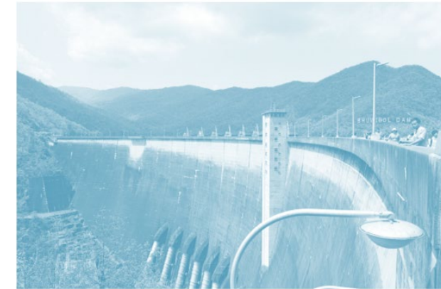
Bhumibol Dam in Tak province, Thailand
