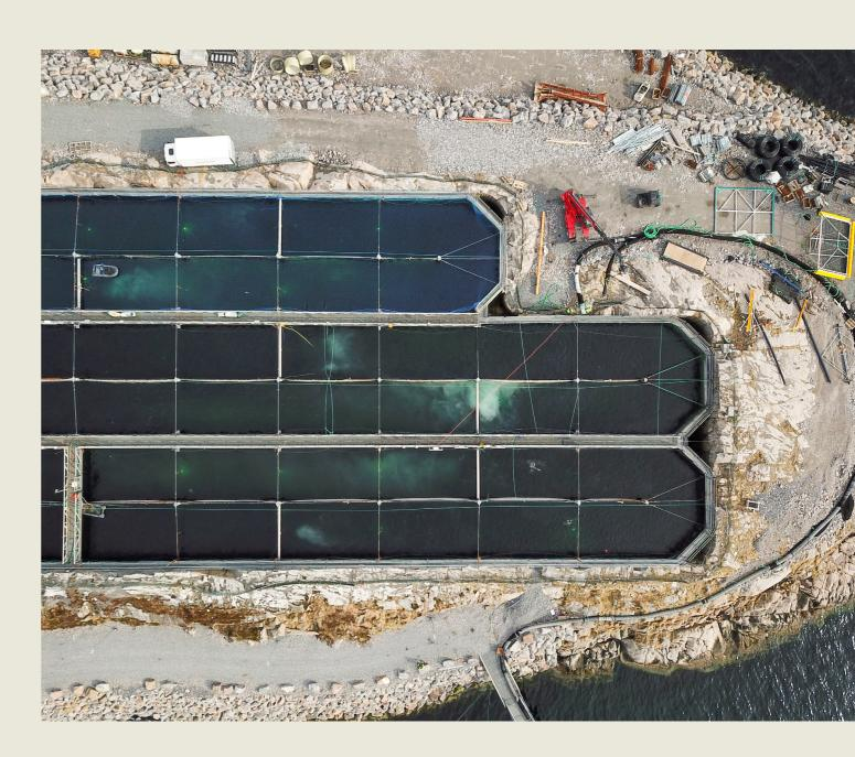
Mechanical, electrical and plumbing work continued throughout the quarter. Casting of the walls of basin C is complete, and casting of the partitions is in its final phase. The walkways over the drainage channel and into the production basin are complete, and installation of walkways over the production basin is on-going.
