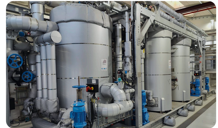
THP system under five-year servicing agreement at Damhusåen WWTP in Copenhagen, Denmark
