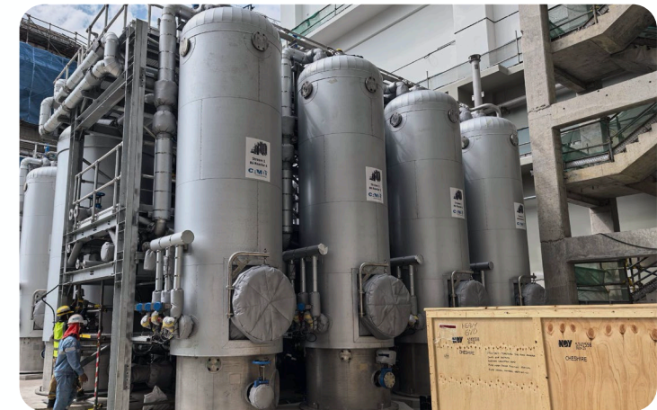
THP systems installed at PUB's Tuas water reclamation plant in Singapore
