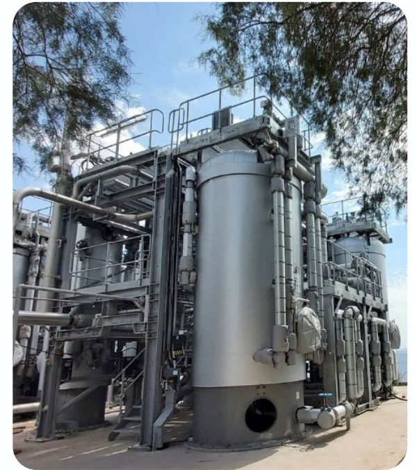
THP systems operating before dryers at the Psytalia wastewater treatment plant in Athens, Greece
