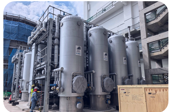
THP systems installed at Tuas in Singapore
