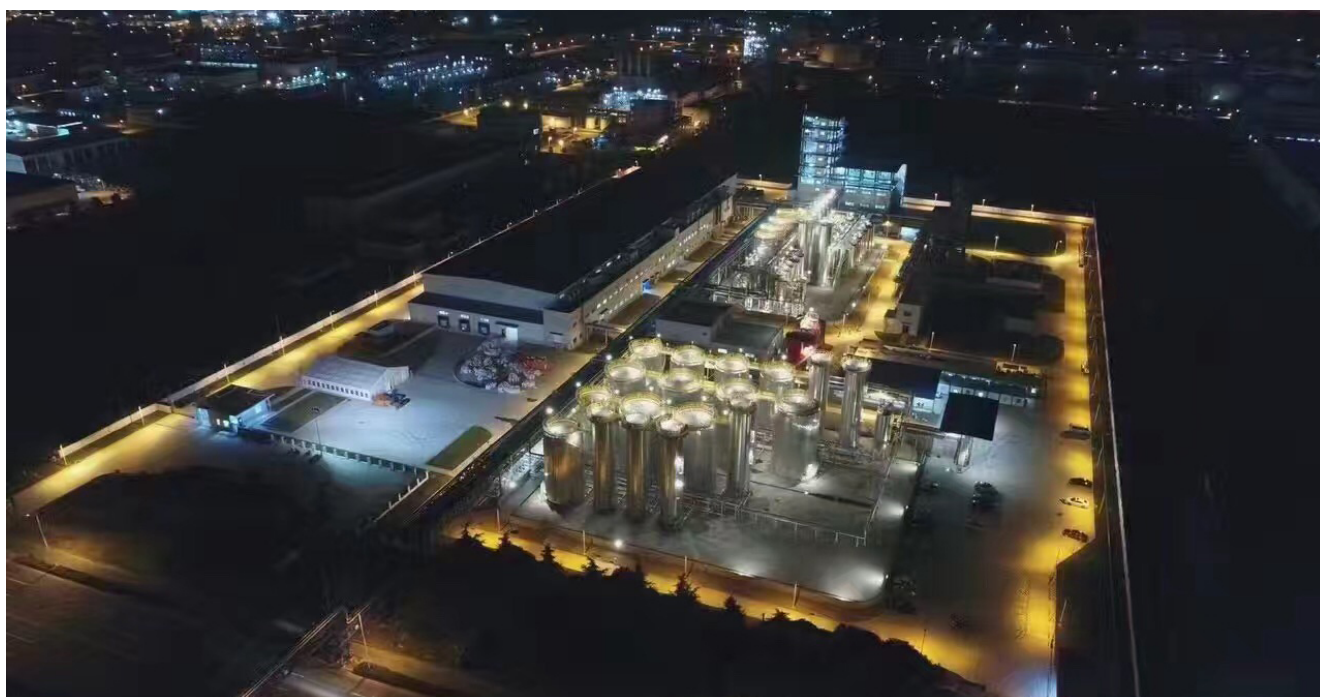
AAK's production facility in Zhangjiagang, China.
