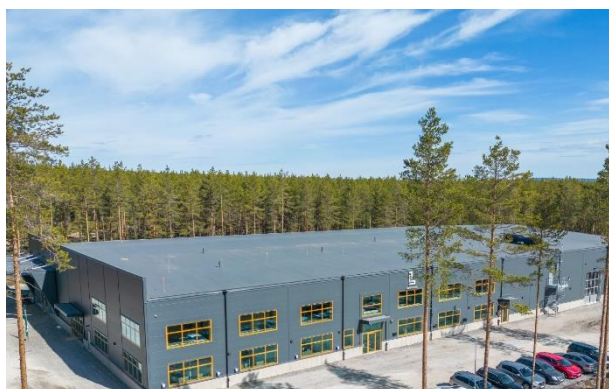
The property Vivsta 13:92 in Timrå, which was completed in 2023
