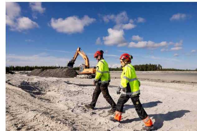
Picture: Sustainability experts on their regular inspection tour at Tailings Management Facility
