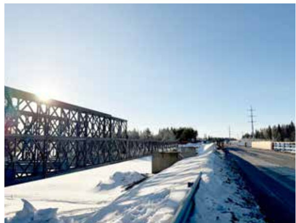
The Autio bridge.
