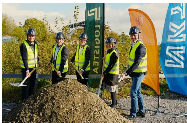
Ground was broken for the project in Alingsås on 10 October 2023
