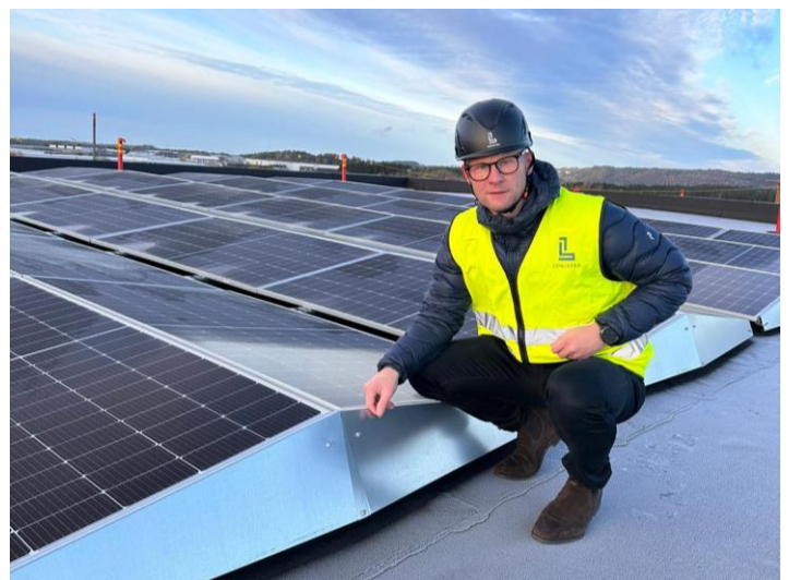
Installation of solar cells on the property Vindan 1 in Borås
