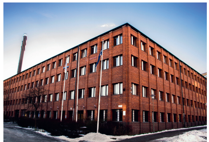
Vincero Fastigheter's property at Instrumentvägen 29-31 in Stockholm consists of offices and storage space.
