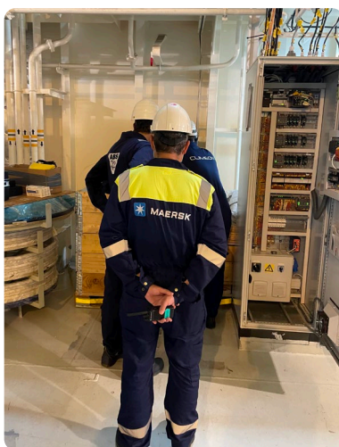
Conducting safety system tests on Climeon equipment onboard Maersk vessel.
