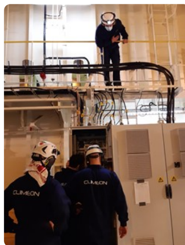
Climeon Team finalizing work on HP System electrical cabinets
