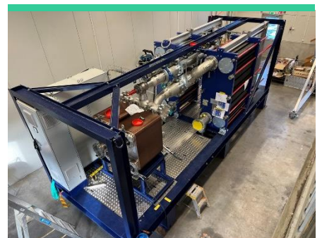
Below: Construction work of the new HeatPower 300 test module.
