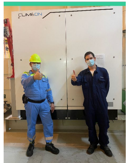
Above: Climeon engineer onboard Maersk vessel.
