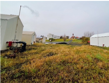
Varmaorka power and district heating plant in Reykholt, Iceland.
